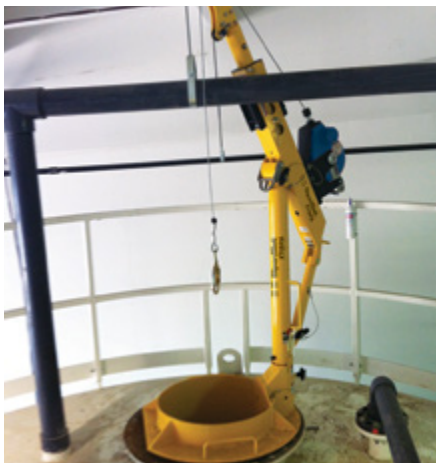
USA2217-05 - Ladder Adapter for Manhole Cover
