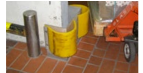
Stainless steel collision protection [food industry]
