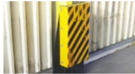
Collision protection for building supports
